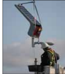
Lift into place
