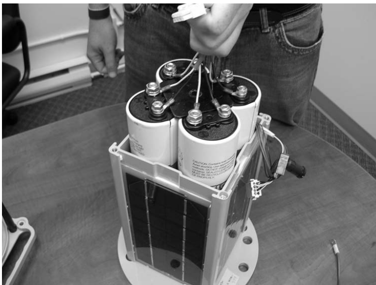
Figure 11-7: Removing the Batteries
