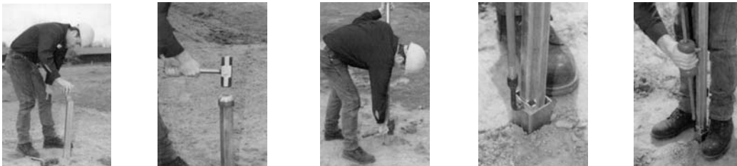
Figure 3: Nex® Sign Support System Installation
